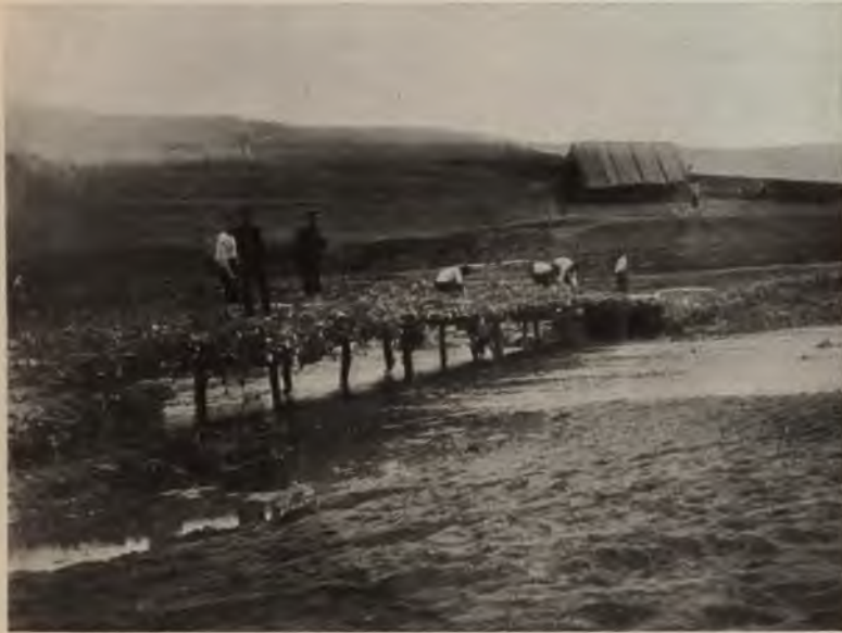
Japanese soldiers erecting temporary bridge.
